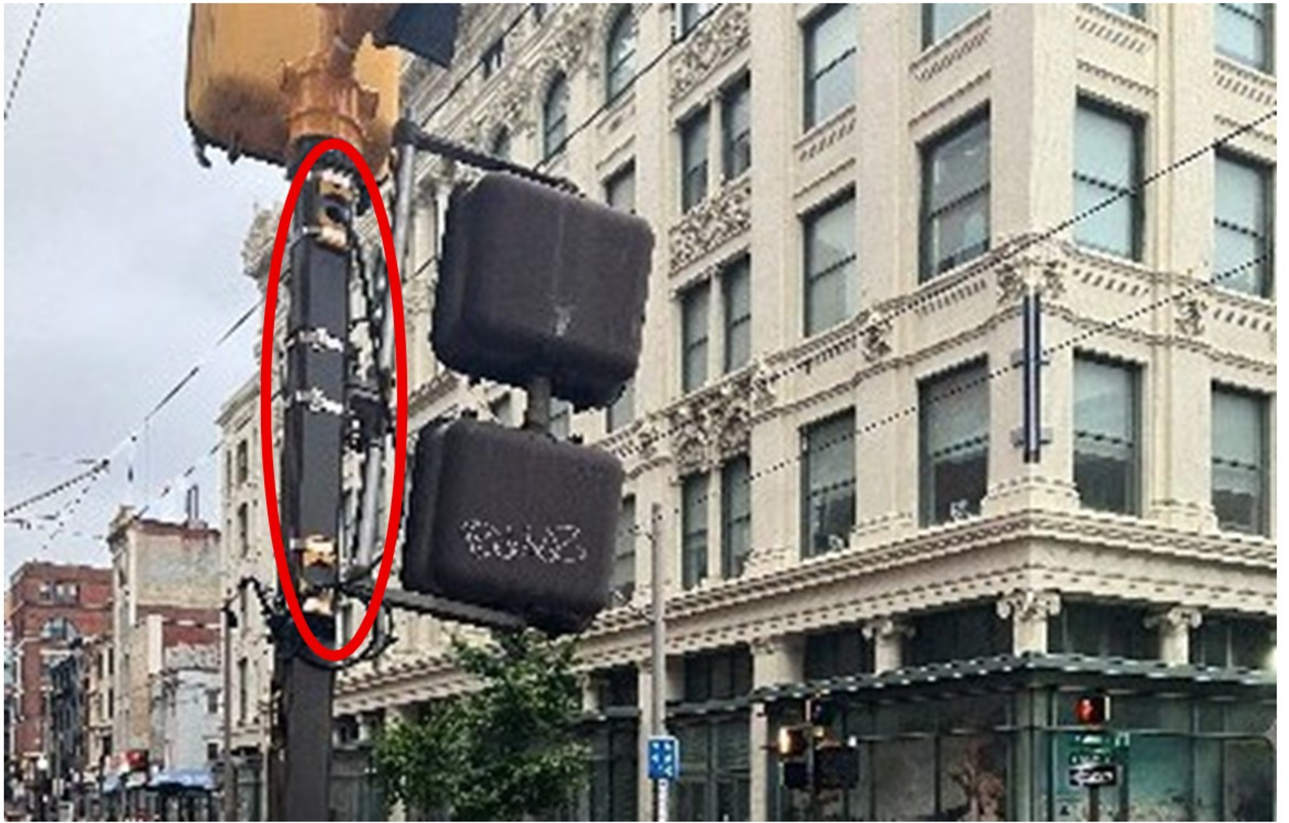
Figure 1 – Missing train coming sign at Howard and Lexington streets.
