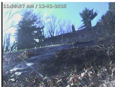
Showing front of house. Entry point snake line in front yard.
