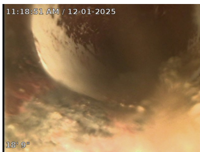
Change in line from cast-iron to PVC.
