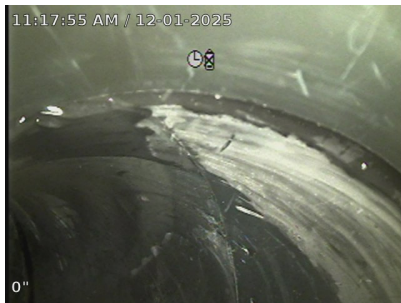
Beginning of cleanout.
