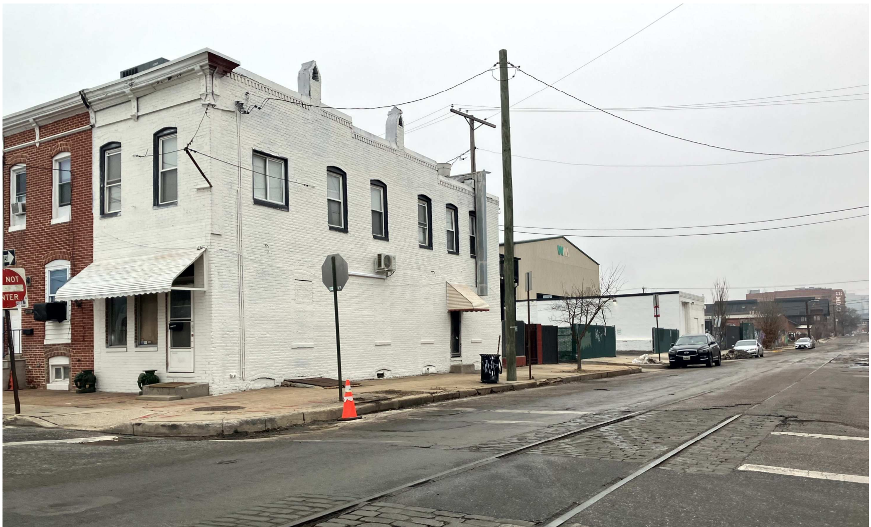
Cone in street At corner of 1537 Bush St on 2/18/26 at 9:11 AM
