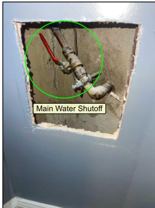
16. Front of the basement
