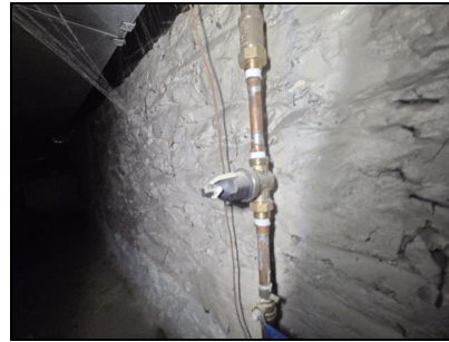
Pressure regulator sometimes referred to as a pressure reducing valve.
