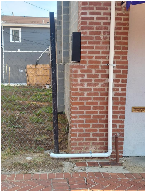
2-1/4" PVC Downspout installed on July 4 th 2026.
