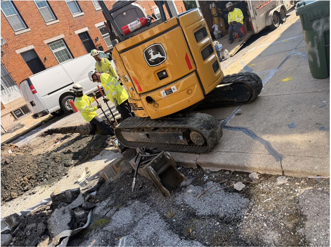
Photo 1 - Heavy tracked machinery positioned directly on the sidewalk at the edge of the excavation.
