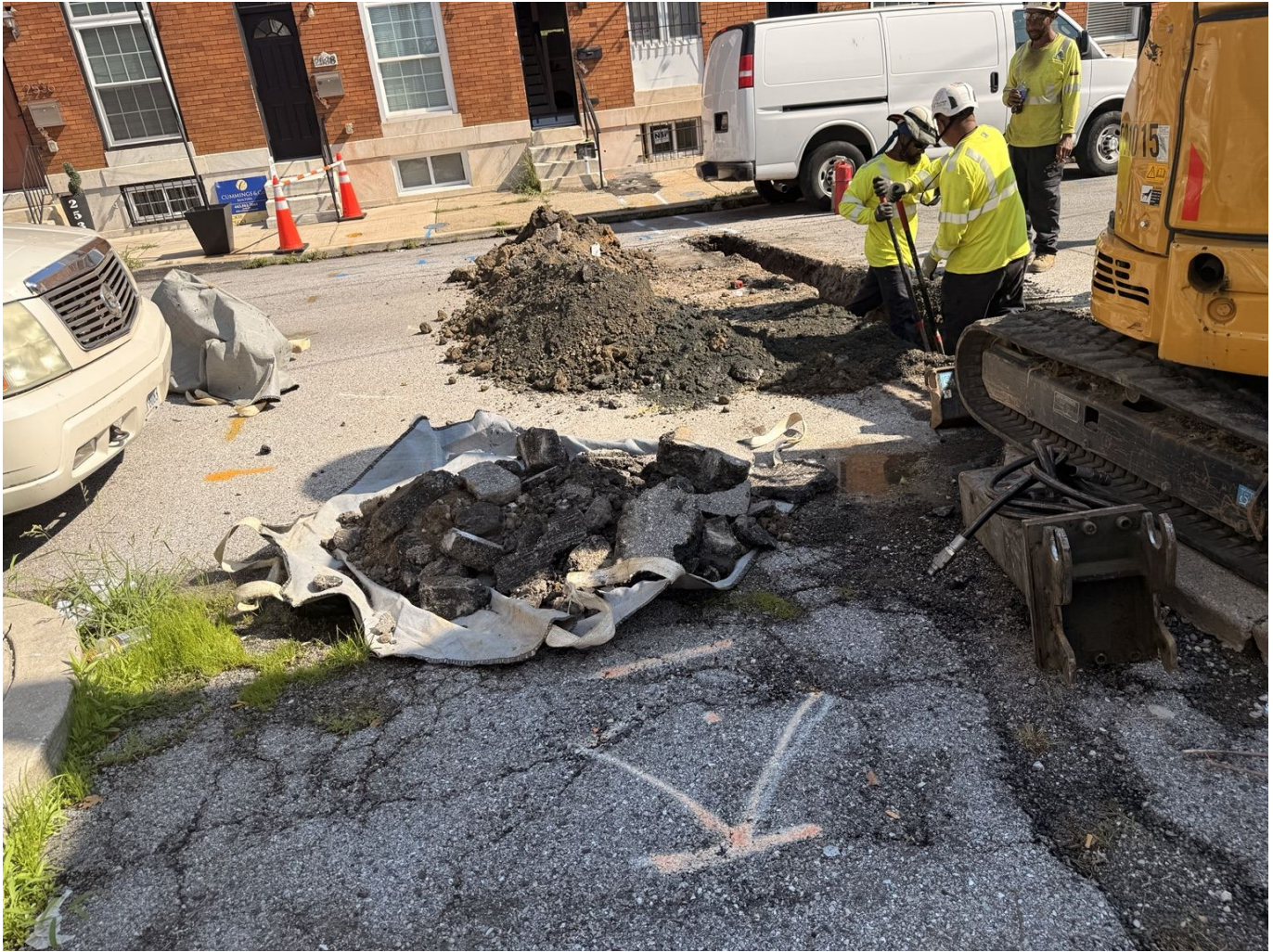
Photo 4 - Wider view of the street excavation, removed pavement, workers, and heavy machinery.
