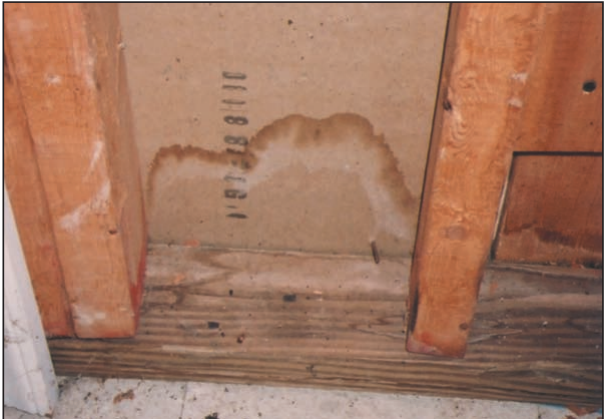
Water stain on a basement wall — locate and fix the source of the water promptly.
