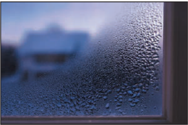
Condensation on the inside of a window-pane.
