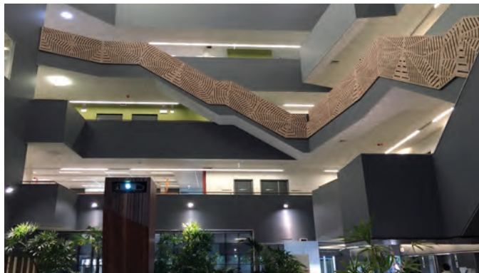
Project QUT Kelvin Grove Partnering Office Designer Bureau Proberts Architects Product Bhushan 2D Perforated Screen in Reatec with ply core
