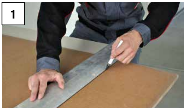
Measure and mark cutting line
