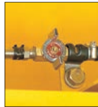
Fuel drain valve
