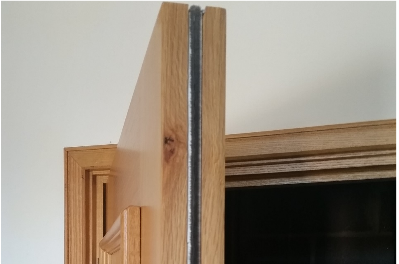
Combined intumescent strip-seal (image courtesy of Golden Thread Fire Delay)
