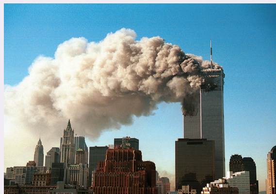
Shortly before their collapse, smoke billows from the World Trade Center's 'Twin Towers' in New York City, which were struck by two hijacked airliners on 11 September 2001
