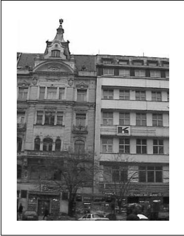
Figure 1.8 ● Two listed buildings.
