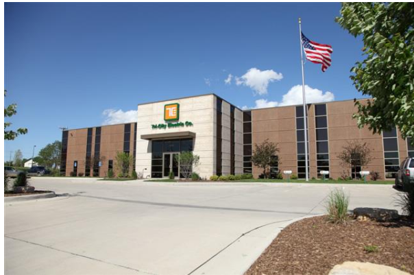
Source: TriCity Electric
