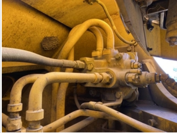
Appearance of Hydraulic Lines / Fittings Photos
