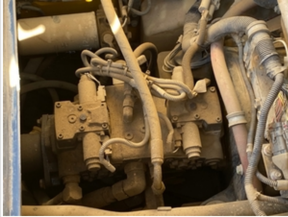
Appearance of Hydraulic Lines / Fittings Photos
