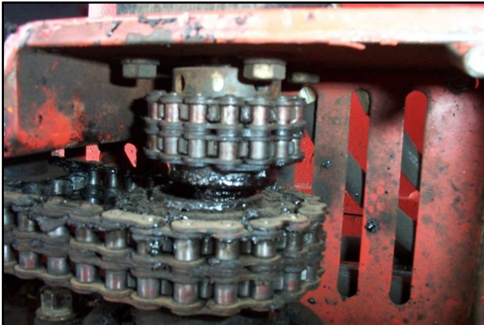
Fig. 6-3 Agitator and Pump Shaft Alignment
