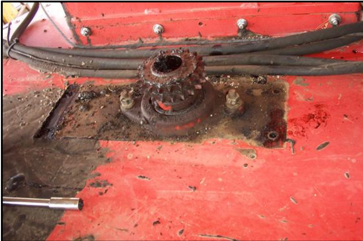
Fig. 6-4 Removal of Motor Mount Assembly
