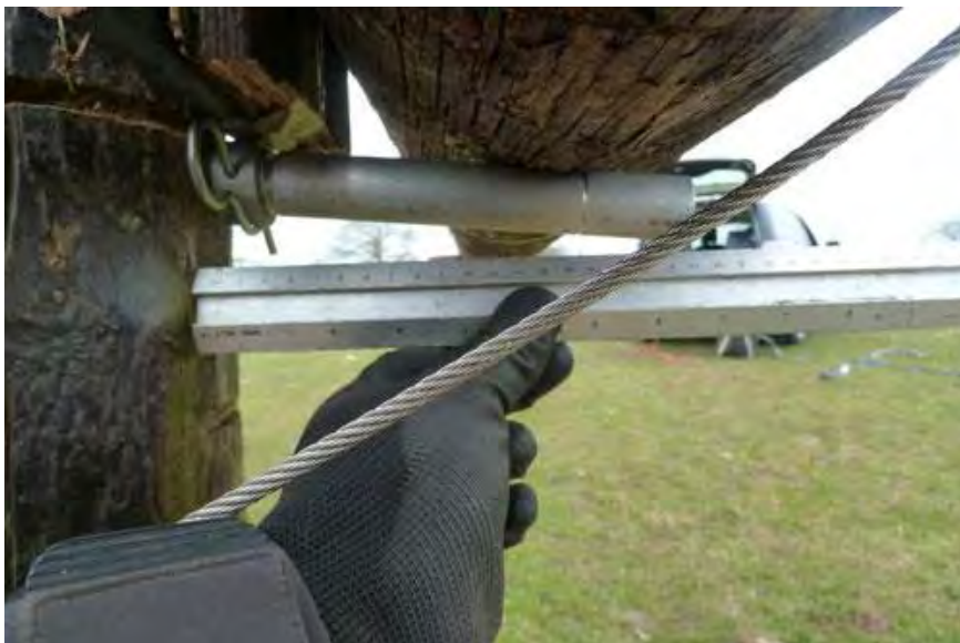
Figure 8 – A pin indicating fatigue by bending which is clearly visible
