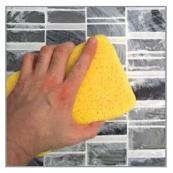
Allow grout to harden for about 20 to 30 minutes. Using a slightly damped cellulose sponge, loosen up all excess grout over the tile with a circular motion. Do not add water before all is well loosened up.
