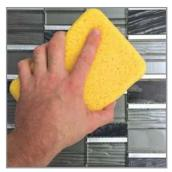
Slightly moisten tile surface with a damp sponge just before application to help with spreading the grout. **Note:** Working time and ease-in-cleanup can be dramatically extended (for up to 2 hours) when using PROMA'S PRO GROUT™ EASE.
