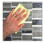
Wait at least 15-30 minutes before removing the final haze from the tile or stone surface with a slightly dampened white scrubbing pad or a microfiber towel.
