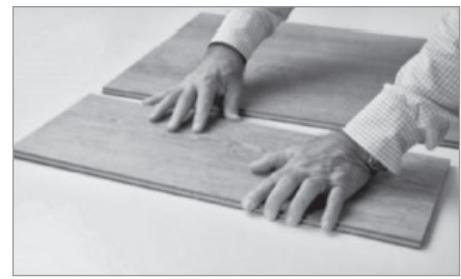
4. To disengage on the short side, slide the planks the opposite direction.
