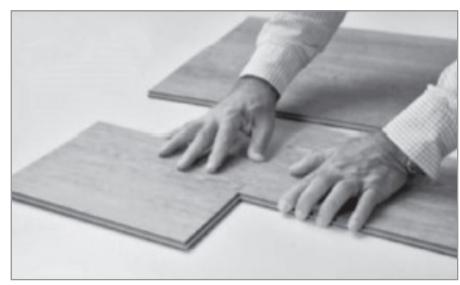
6. Continue sliding until the planks are fully separated.
