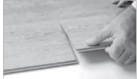
3. Press with your thumb on both ends of the short side.
