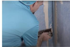
**9.** Fold AlinO Band into half to create a crease for easy installation and install along the vertical (wall to wall) and horizontal (wall to floor) joint with modified thin set mortar.
