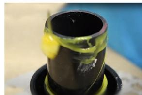
**5.** Take out the cover from pipe outlet and connect AlinO Drain body with pipe outlet by using ABS/PVC glue (may need to add small ABS/PVC pipe if there is any gap between drain connector and pipe outlet).
