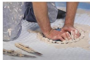
**6.** Install drain body with modified thin set mortar on shower tray. Press the drain body and hold it for a few seconds to properly bond drain connector with pipe outlet. Remove excess mortar on top of the drain flange and cover drain hole with cloth to protect from debris.
