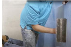
**1.** Install AlinO Seals and AlinO-Gard waterproof membrane on wall by applying modified thin set mortar, using a 3/16 x 3/16 V-Notch trowel. Ensure 2" overlap at every joint, 100% mortar coverage at the back and make sure to remove all air pockets.
