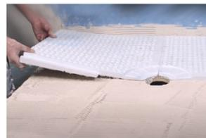
**4.** Clean subfloor with wet cloth and spread modified thin set mortar by using 1/4 x 1/4 V-Notch trowel and position AlinO-Shower Tray (flat side face-down). Ensure 100% mortar coverage on the back of the tray.
