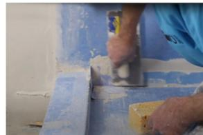
**10.** Install Inside and Outside corners by using modified thin set mortar, and your shower is now waterproof, wait 24 hrs. before tile installation.
