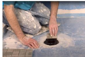
**11.** Install Grate Holder with height adjustable ring/collar by using modified thin set mortar. Adjust grate holder to flush with tile. Once the desired height is achieved, align the grate holder with the grout line through lateral movement, and remove the excess mortar, and continue tiling.
