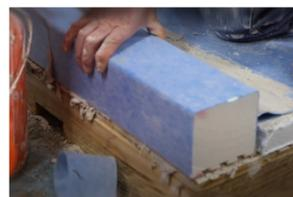
**7.** (Ignore this step for curb-less shower). Measure and cut the shower curb as per requirement. Install Shower Curb using modified thin set mortar. Ensure channel side at the bottom and top sloped side are facing towards the shower.
