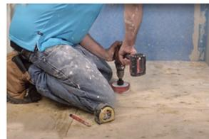
**3.** Position AlinO Shower Tray and mark the subfloor to indicate the position of the hole to access pipe outlet. Remove shower tray and cut a 4-1/2" diameter hole by jig saw or hole-saw and cover drain outlet to protect from debris.
