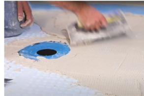
**8.** (Ignore this step if AlinO Gard waterproof membrane is already bonded with tray) Apply modified thin set mortar on the tray using 1/4 x 3/16 V-Notch trowel and install AlinO-Gard waterproof membrane on the tray.
