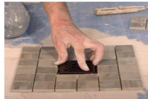
**12.** Snap on stainless steel grate (does not require any screws) and your shower is ready for use.
