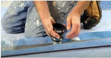
Join AlinO Linear Drain with 2" No Hub Coupler. Measure the distance between drain and the pipe, cut a small piece of 2" pipe to join (if required) by using ABS/PVC solvent. Apply modified thin set mortar on the substrate, and position drain body support and then drain body.
