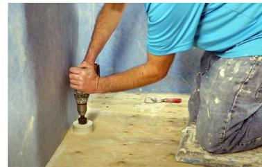
Once location for drain is identified, cut a 3-1/4" to 3.75" hole in the substrate, **Skip step 4, if you are not using AlinO Linear Tray.** **Skip steps 3 & 5, if you are not using AlinO-Gard waterproof membrane.**
