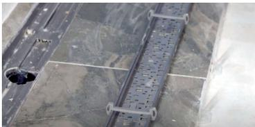
Ensure all plastic clips are attached with the bottom of the grate.
