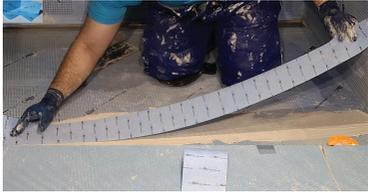
Install all pre-formed inside and outside AlinO-Corners on all corners of the Tray. Cut AlinO Band to length. Fold in half lengthwise to create crease for easy install. Apply modified thin set mortar and press in place using a flat trowel for every horizontal and vertical joints. Use ¼" x 3/16" (6mm x 5mm) V notched trowel.
