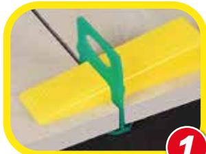
**1** Slide two clips under the tile and into the mortar.
