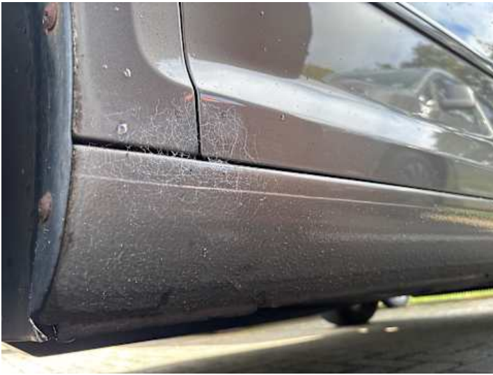
Schweller links (Lackschaden, Rost)
