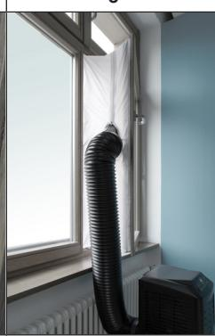
A photograph of the window from a distance. The velcro seal is now fully installed around the perimeter of the window frame. A black flexible exhaust air tube is visible, extending from the window area towards the bottom right corner of the frame. |
