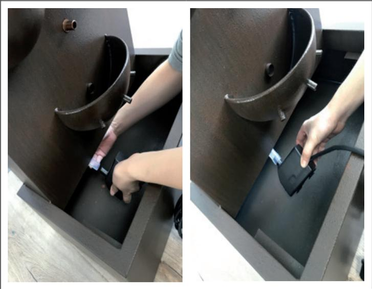
**3: Run the pump cable from the front to the back of the fountain.**
