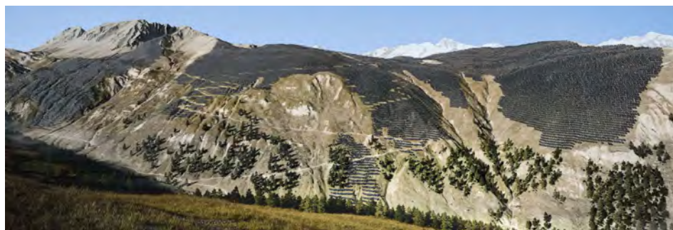
Figure 34 – Grensiols-Solar originally projected at 600GWh over a surface of 6.6km 2 (Ivanova, 2023)
