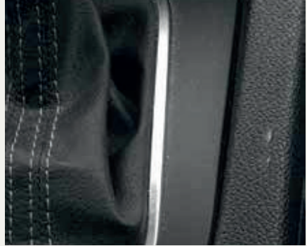
Minor damage to plastic moulding
