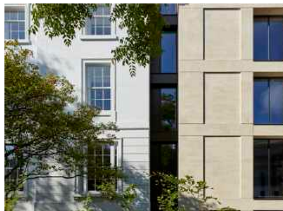
▲ Glazed link between existing & new, One Bayshill Road, Cheltenham
