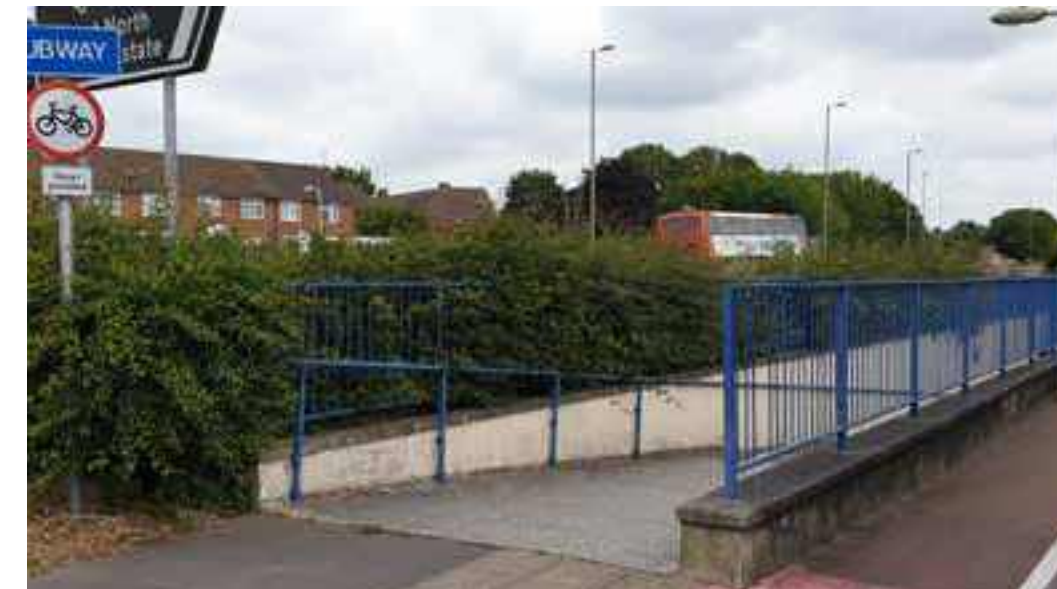
Z1.1.1a Petersfield Rd (B2149) Subway
