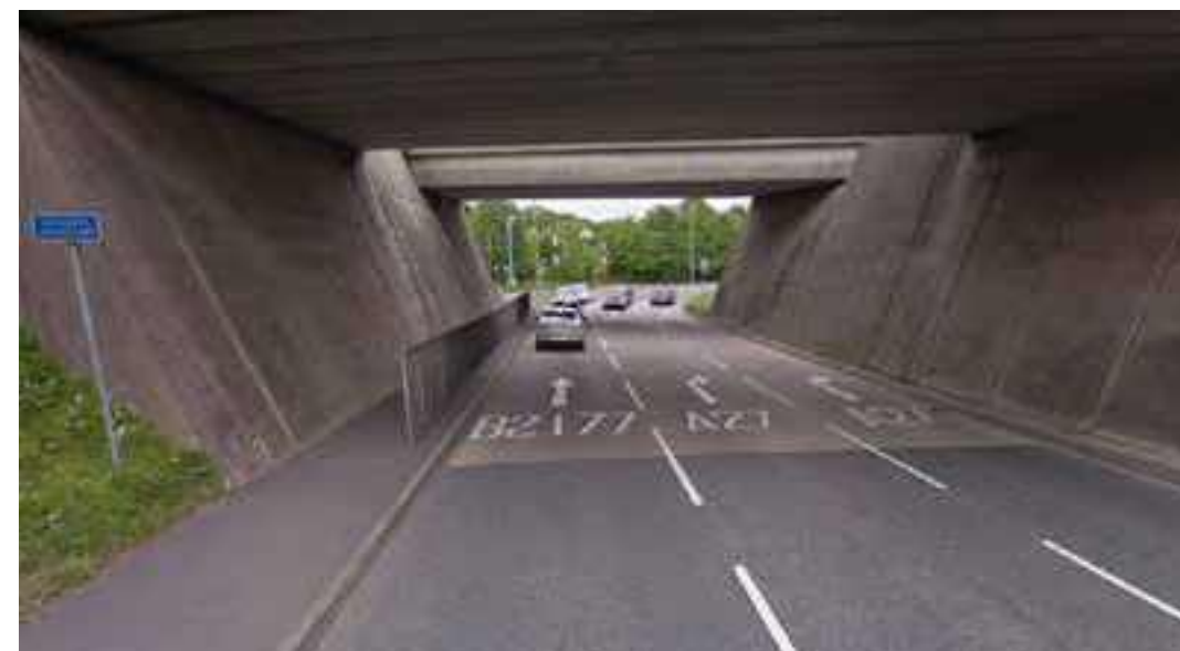
270.2.8 Under the A3(M)
