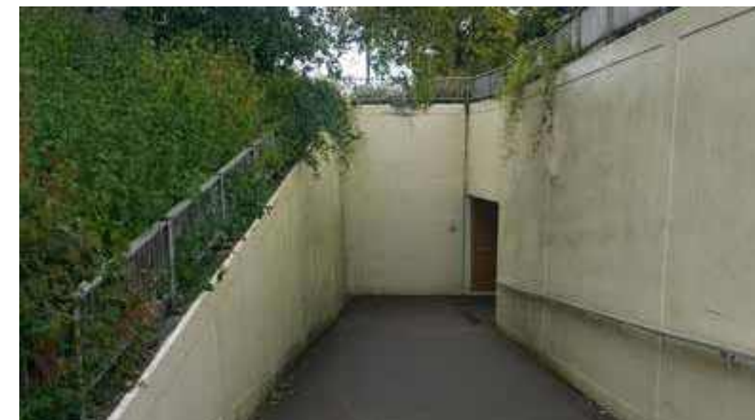
Z5.3.2b Underpass beneath Maurepas Way
