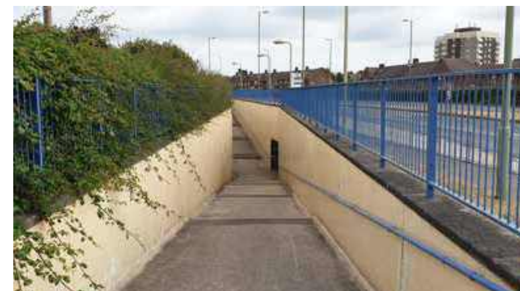
Z1.1.1c Petersfield Rd (B2149) Subway
