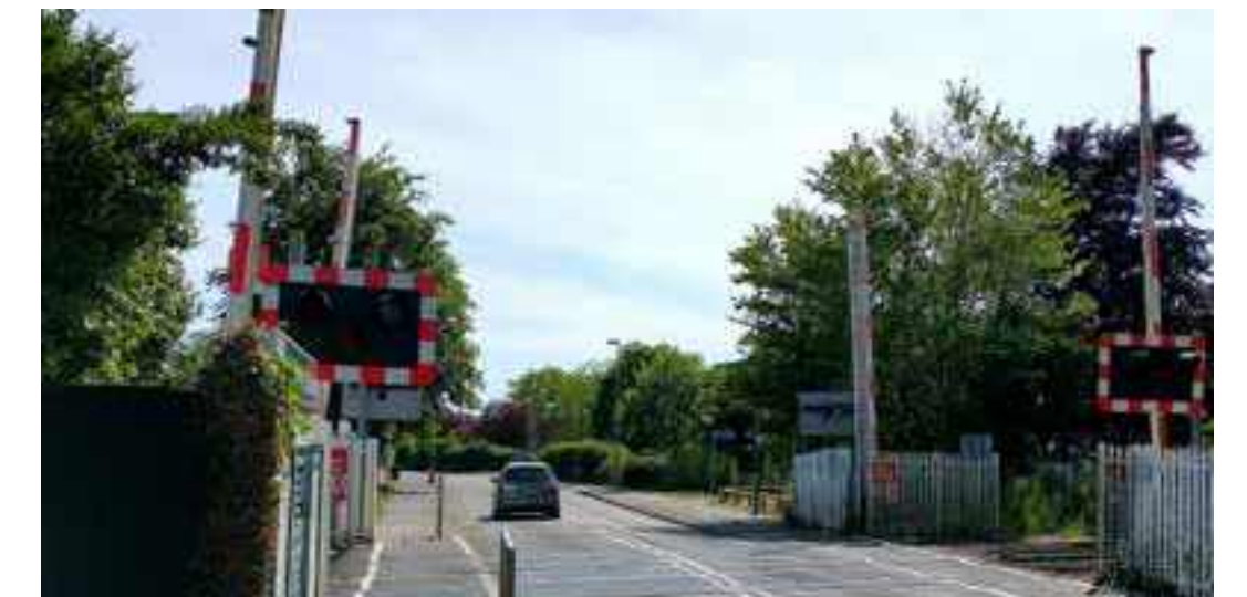
372.1.2 Warblington Train Station Level Crossing (Southleigh Road)
