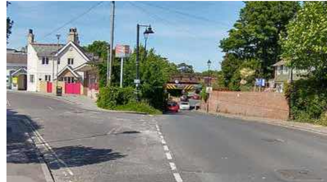
373.1.6 Emsworth Station/railway underpass
