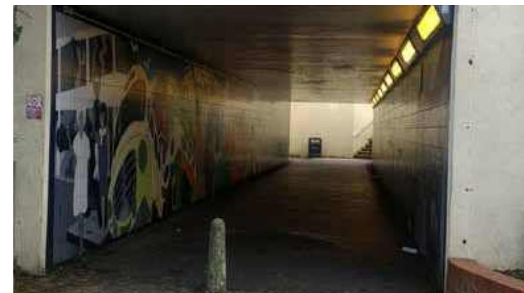
Z5.4.1b Hambledon Road underpass
