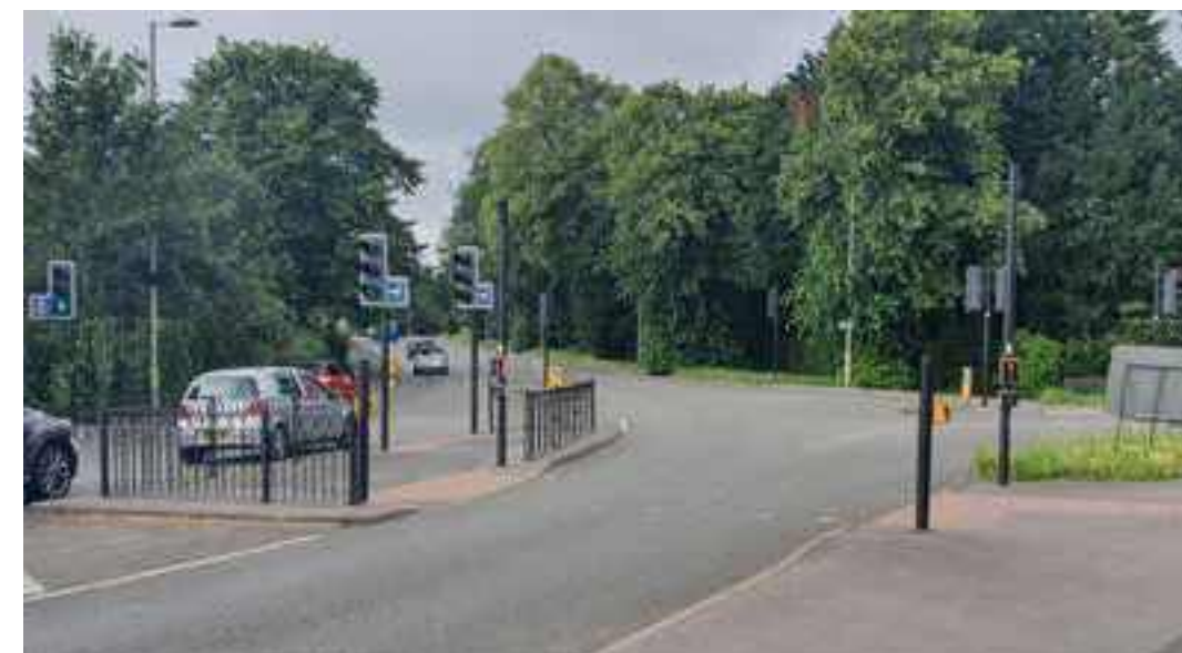
275.1.7 Bedhampton Road/Hulbert Road
