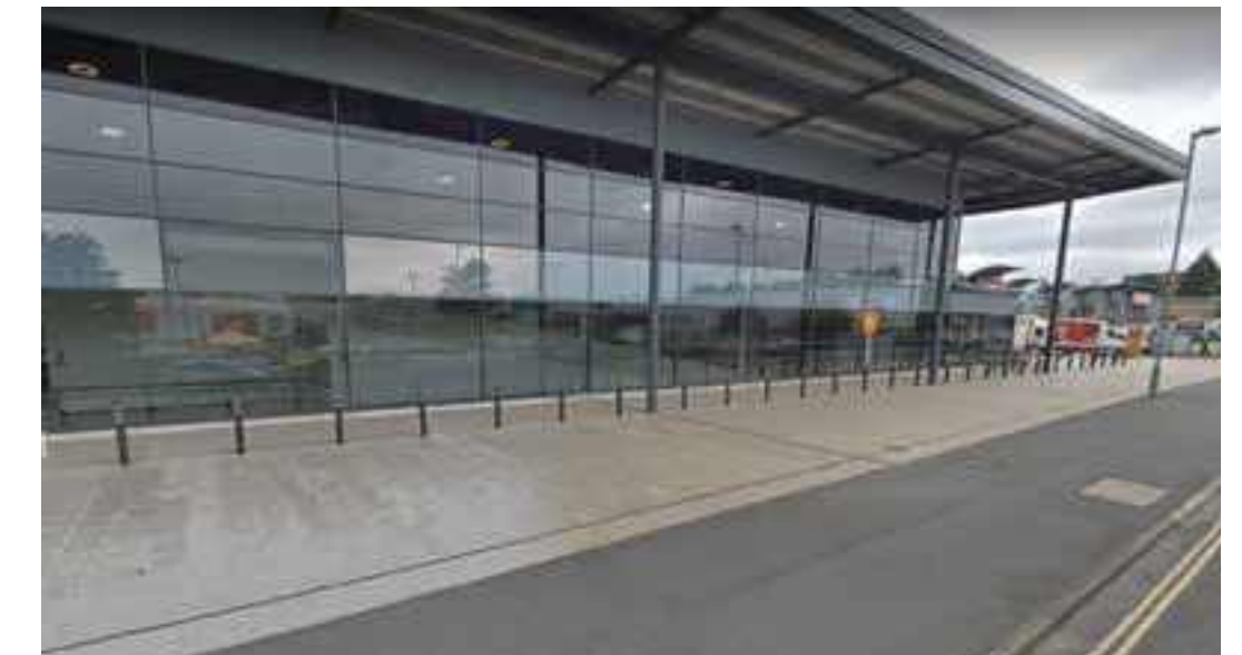
Z5.5.4 Footway along Hambledon Road
