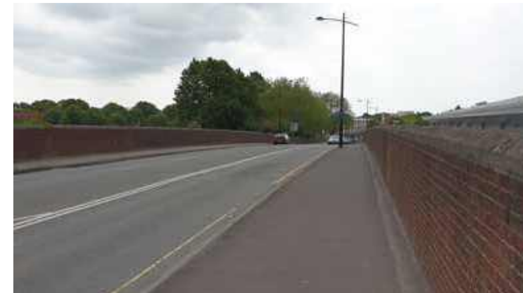
Z1.3.1 Park Road North
