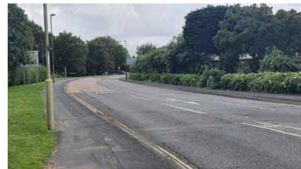
Z1.2.3 Elmleigh Road east of roundabout
