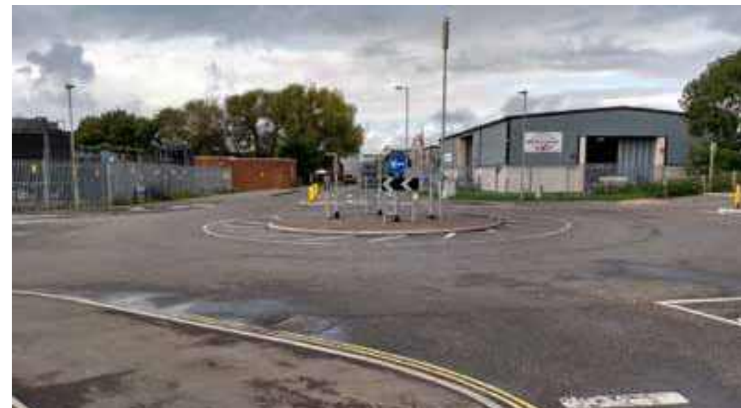
270.2.5 Harts Farm Way/Brockhampton Road
