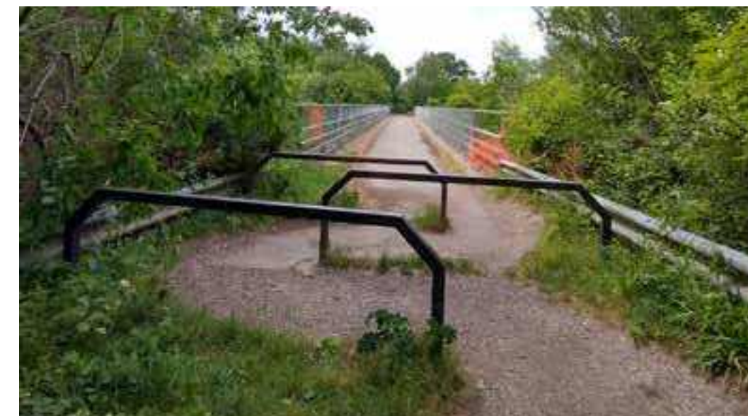
362.2.3 Bridge over A3(M)
