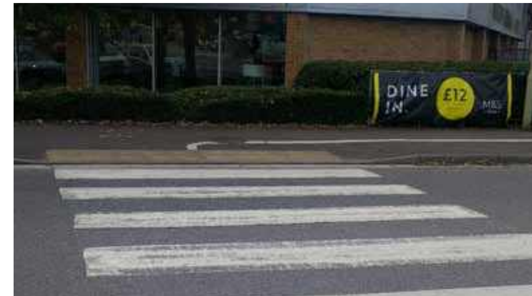
Z5.5.1 Pedestrian crossing on Hambledon Road
