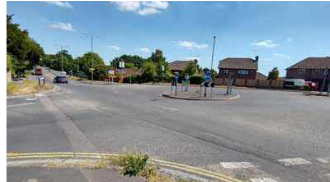
275.1.4 Bedhampton Road Roundabout
