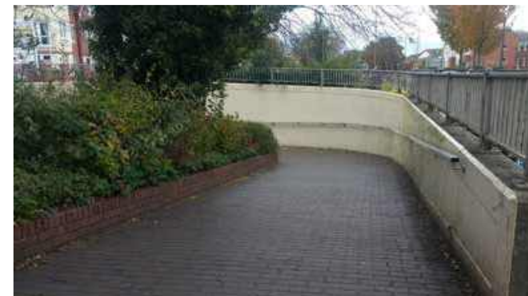
Z5.3.2a Underpass beneath Maurepas Way
