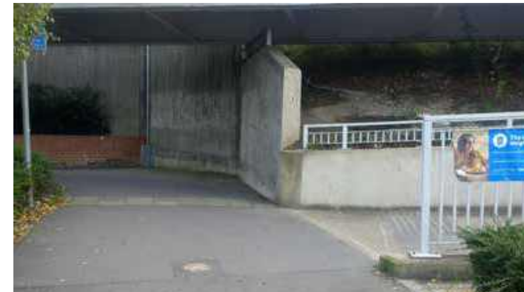
Z5.4.1a Access to Hambledon Road underpass
