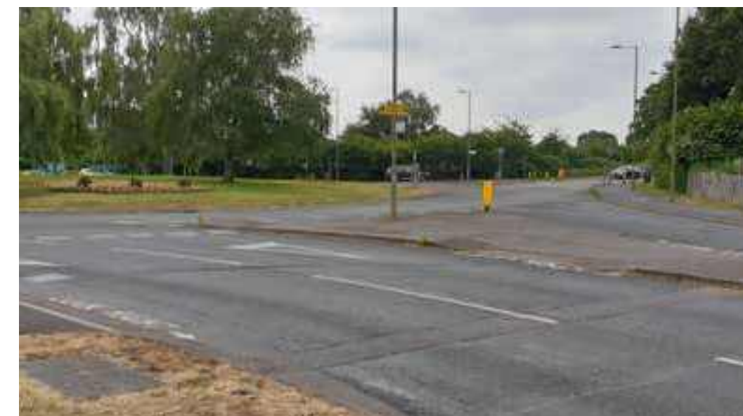
Z1.2.2 New Road west of roundabout
