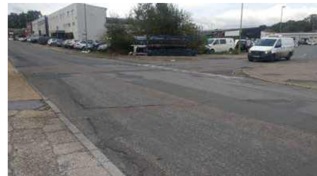
Z5.6.1 Aston Road and side street
