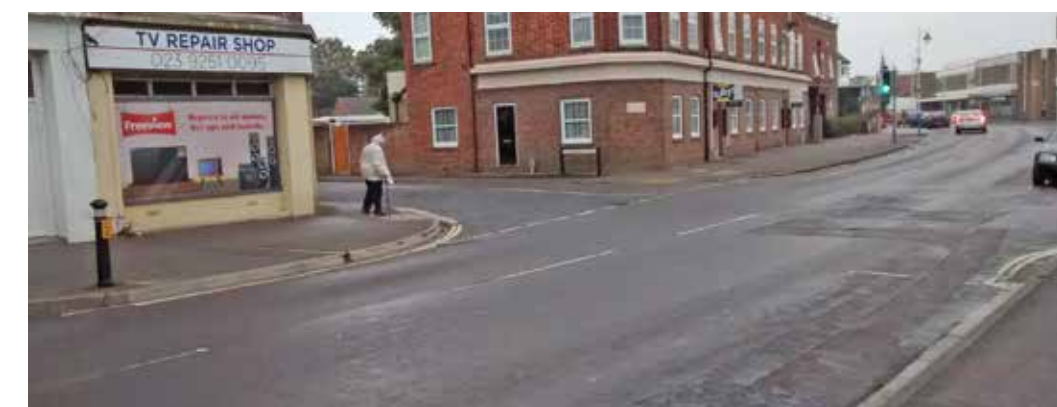
Z3.3.2 Stoke Road typical junction with side street
