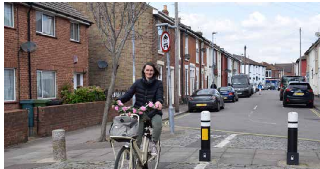
Point closure with removable bollards – Portsmouth City Region
