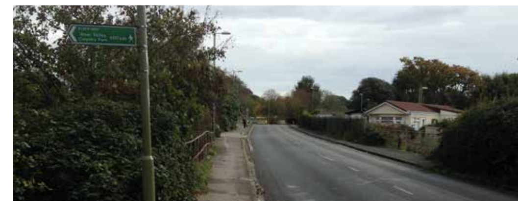
265.4.3 River Alver bridge
