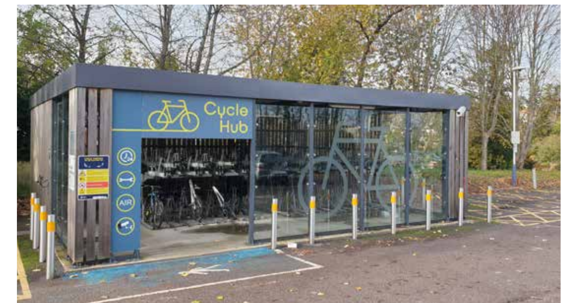
An example of cycle hub parking facilities – Winchester Train Station
