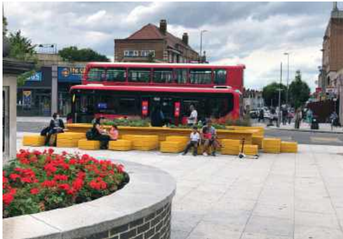
2 Existing public realm around Albert Crescent.
