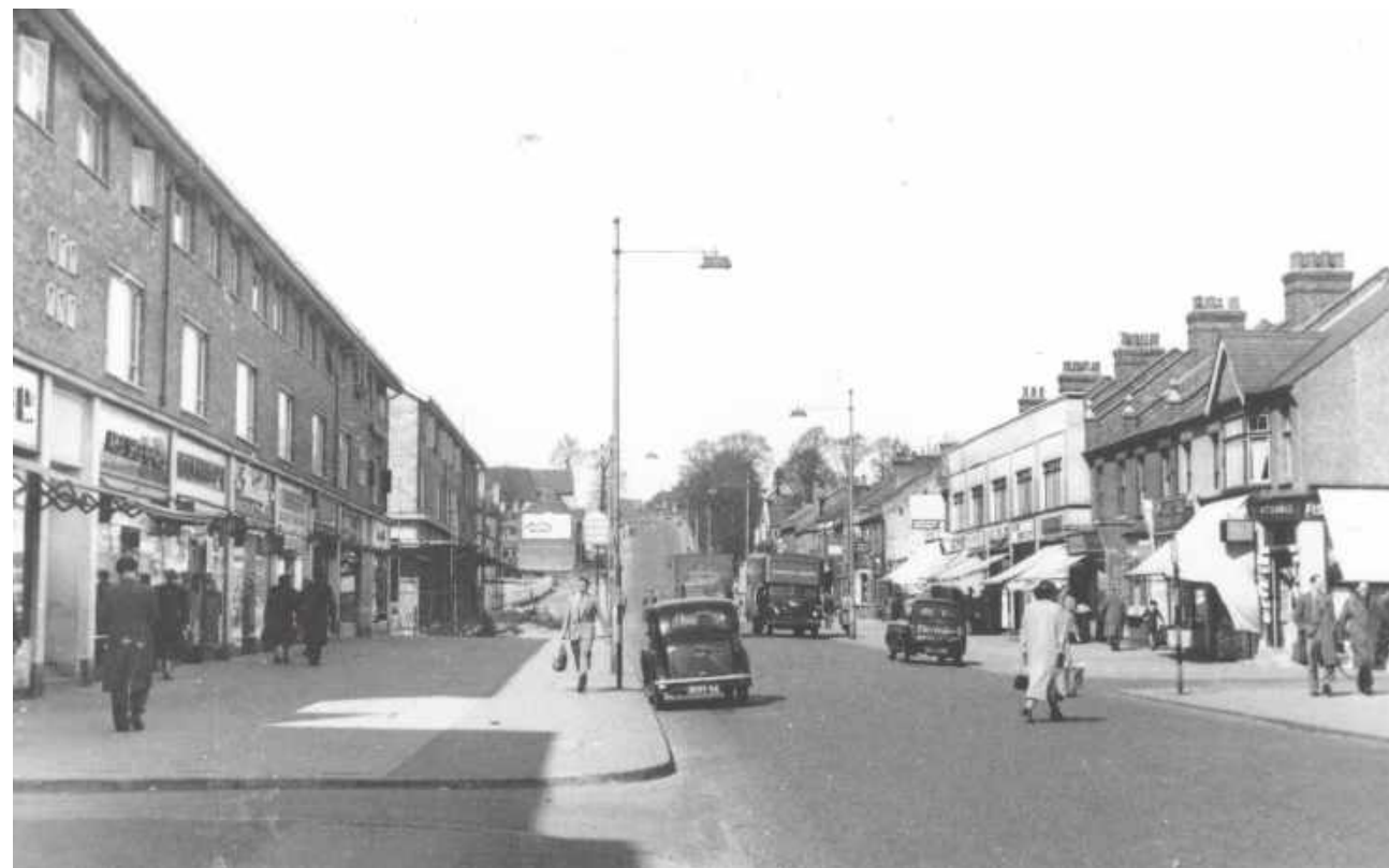
1955 Photograph looking north along Old Church Road showing Churchill Terrace buildings under construction.
