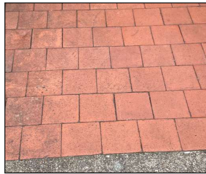
5. Coloured floor tiles as seen on Russell Avenue
