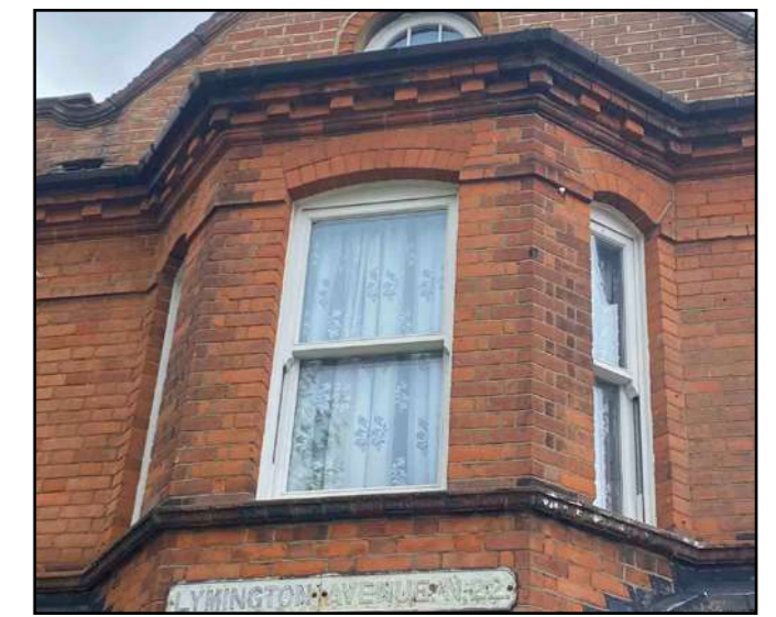
8. Angled brick piers with vertical windows as seen on Lymington Avenue
