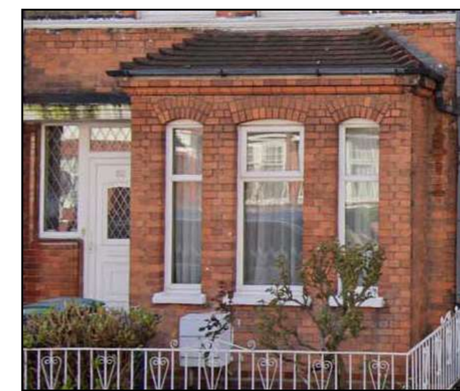
3. Triple windows with a larger central window as seen on Russell Avenue
