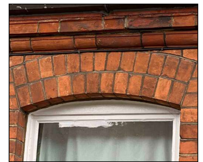
4. Brick on end above windows as seen on Lymington Avenue
