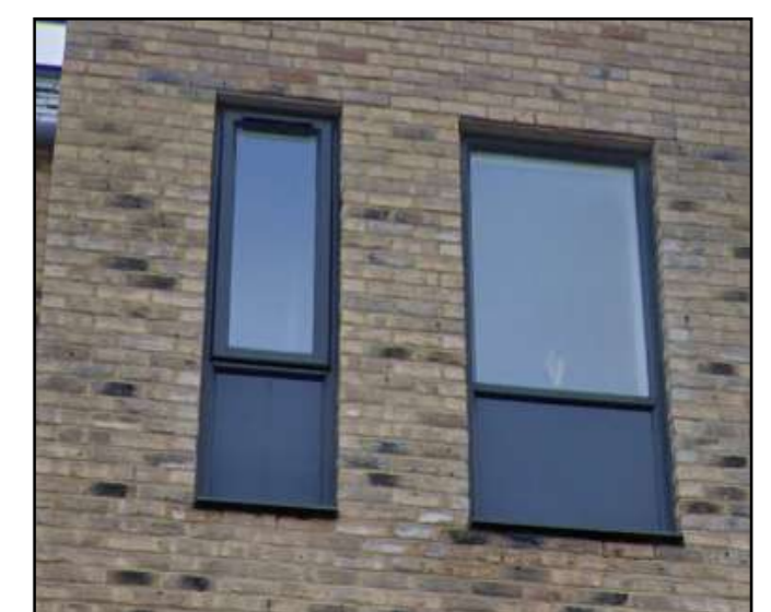
12. Aluminium infill panel below windows
