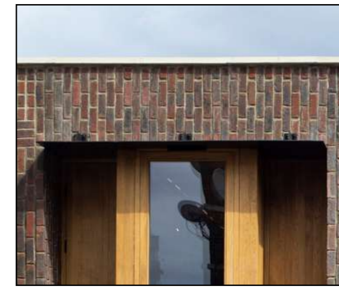
7. Solar shading above windows
