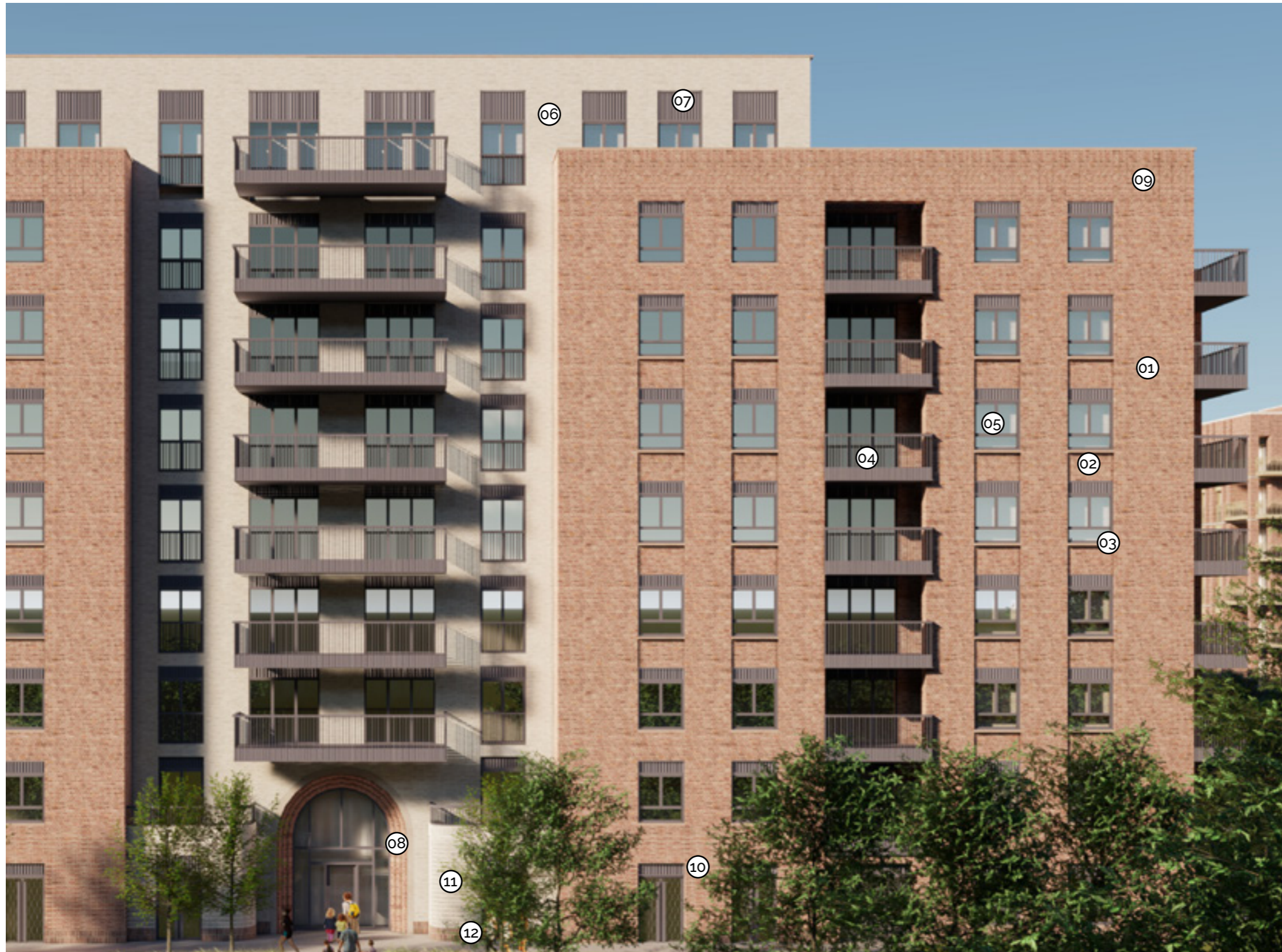
Block B/C West Elevation Bay
