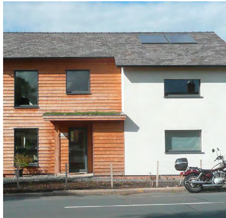
Image 41: 41 Rooftop Solar Thermal Panels at Wairoonga
