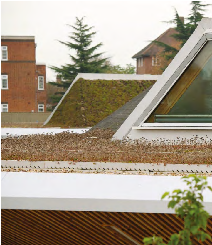
56 Image 56: Green Roof, Architype
