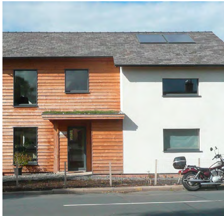
Image 41: 41 Rooftop Solar Thermal Panels at Wairoonga
