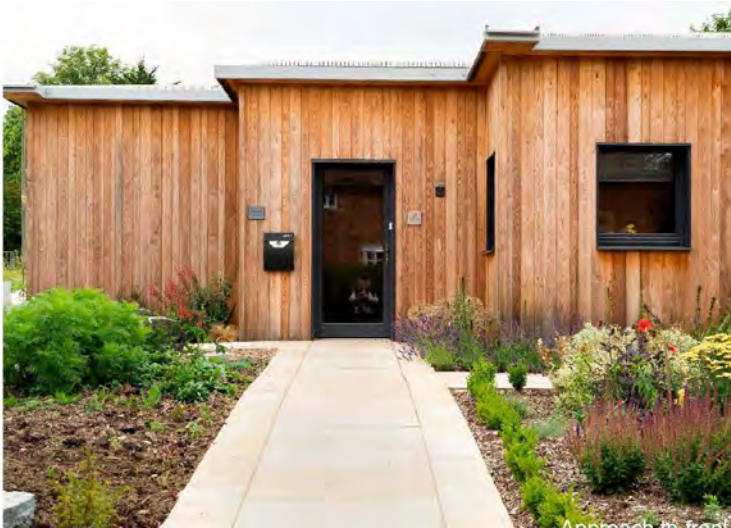
▲ Image 106: Entrance, Passivhaus Trust
