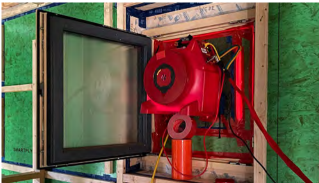
74 Image 74: Air test during construction
