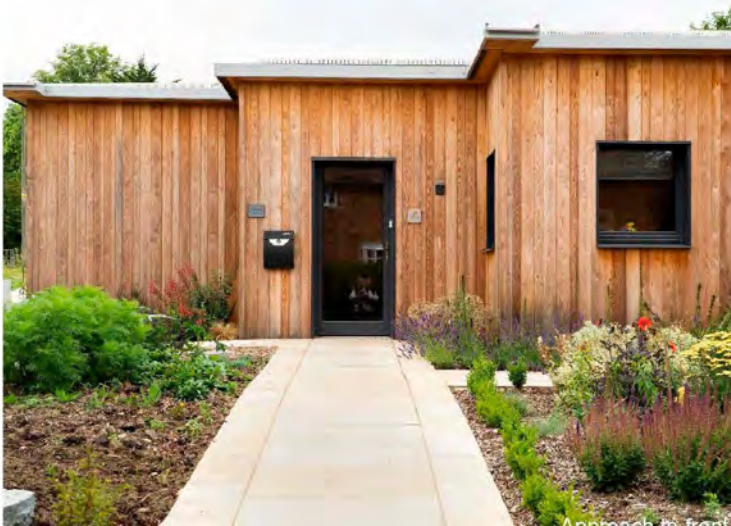
▲ Image 106: Entrance, Passivhaus Trust
