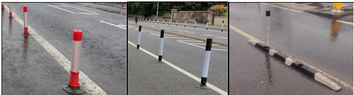
Fig 1: Types of temporary traffic management trialled on A77 (l-r); red & white flexi-cylinder (Fenwick Road), Marshall's swing wand bollard black 1000 (Ayr Road), Rediweld Greenwich Wand Orca (Ayr Road)
