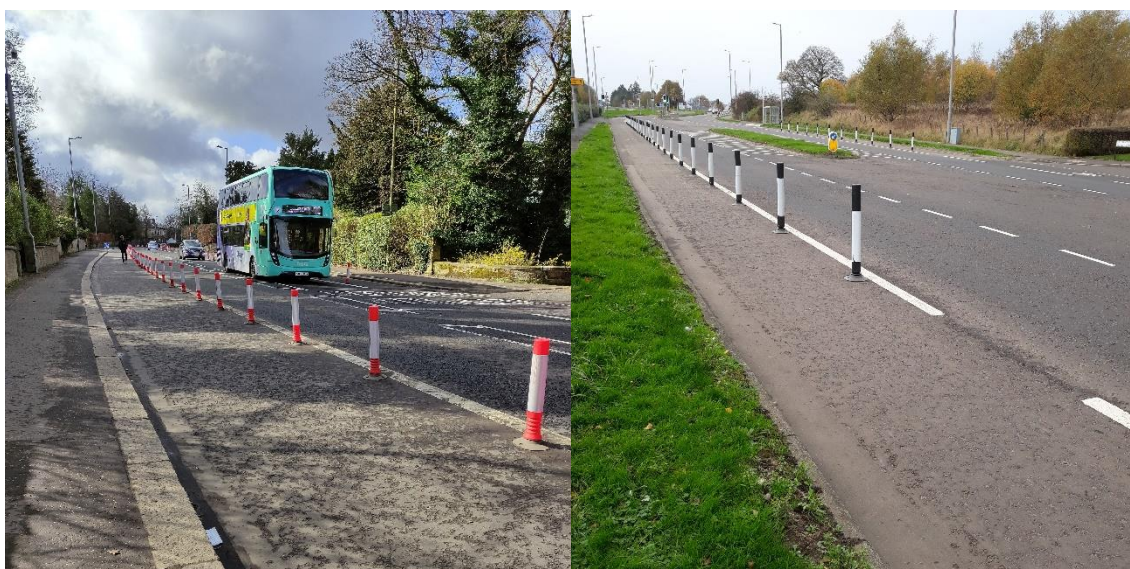
Fig 1: View of typical light segregation adopted along Fenwick Road (left) and Ayr Road (right)
