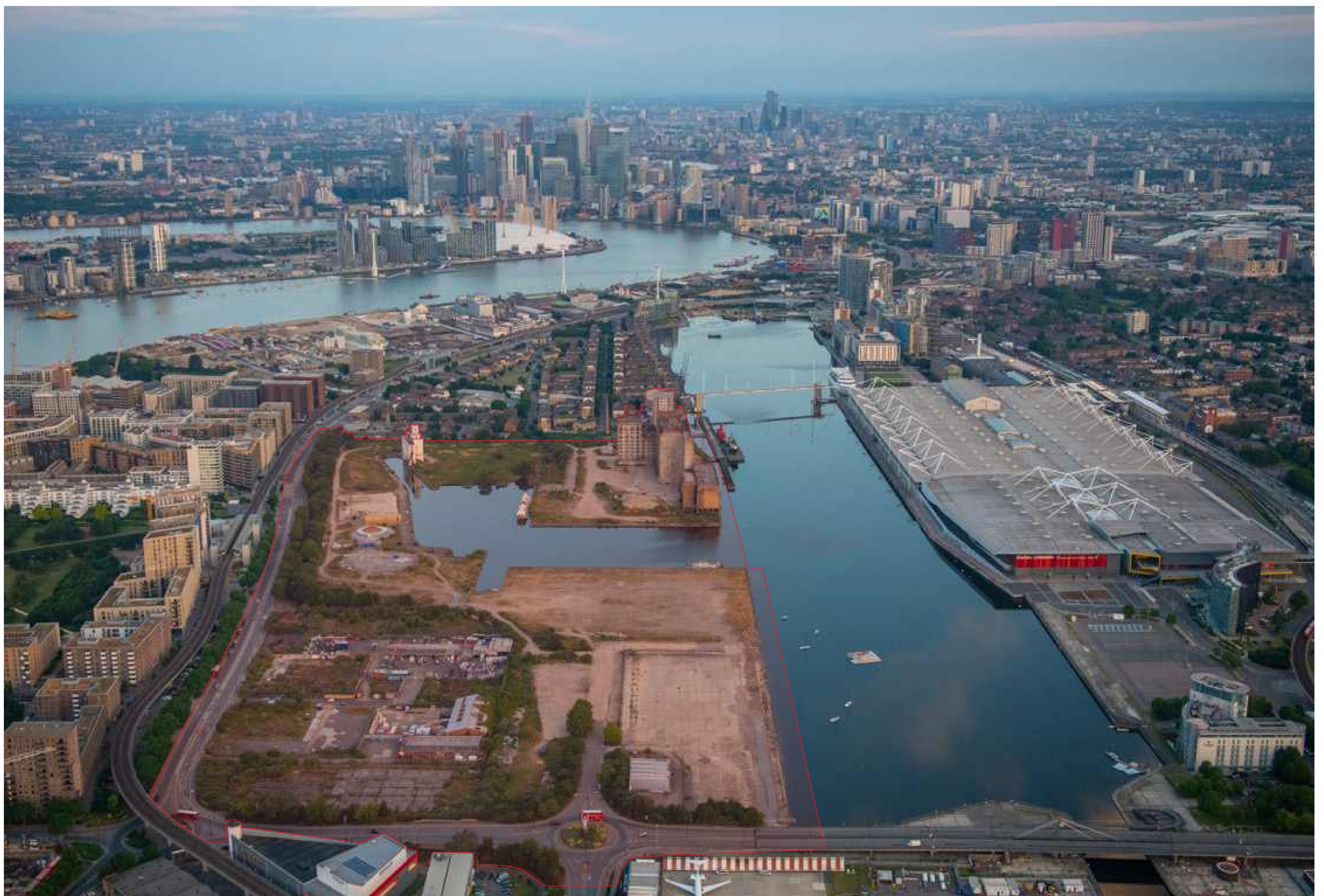
This birds-eye view shows the Silvertown site (outlined) by the Royal Victoria Dock and opposite the ExCeL. The Greenwich O2 and Canary Wharf can be seen in the background.
