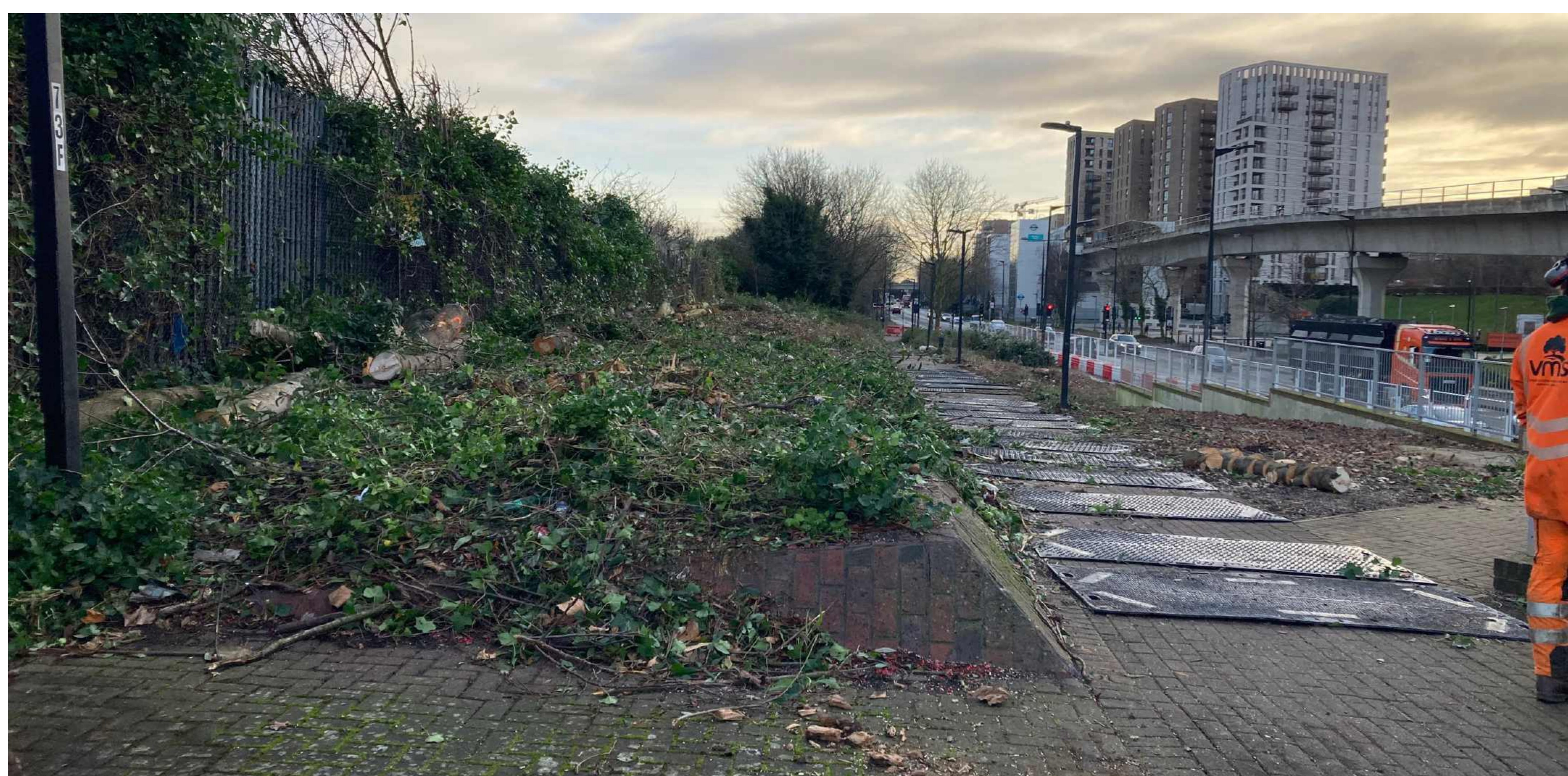
The image above shows some of the trees that have been removed along North Woolwich Road
