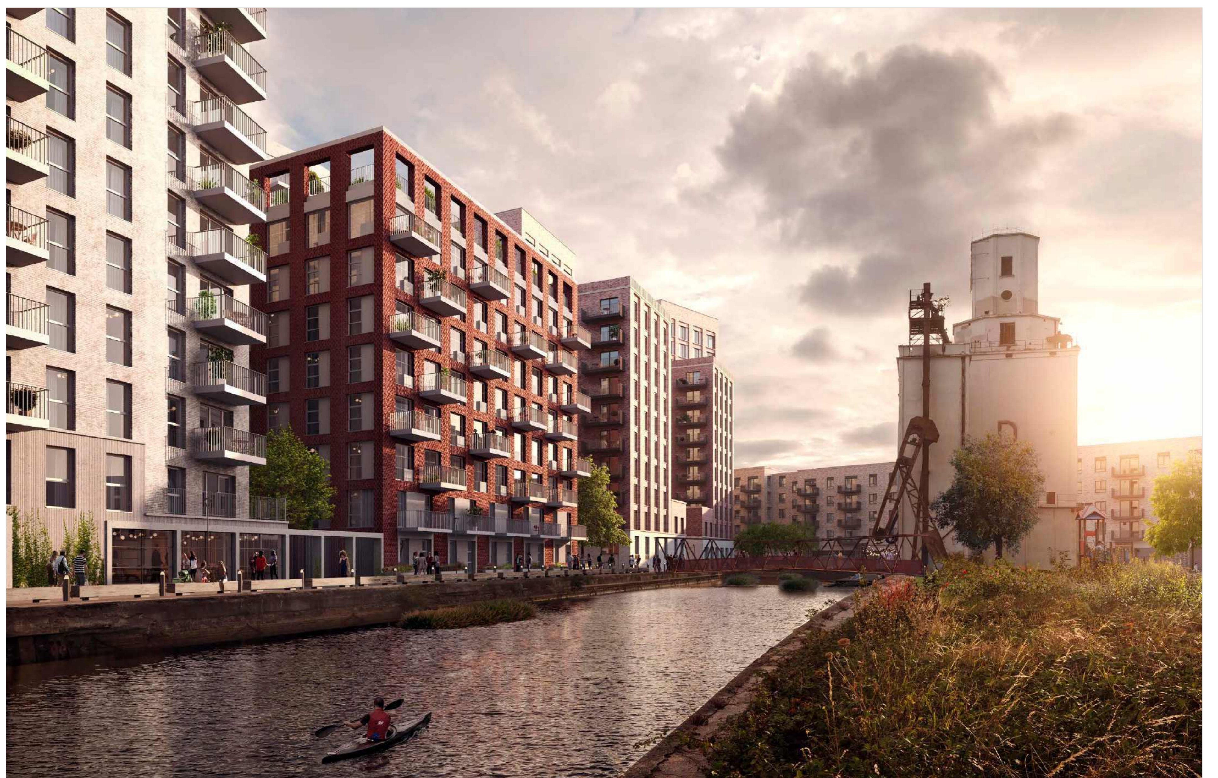
This Computer Generated Image (CGI) shows how the first buildings in Phase 1 may look.
