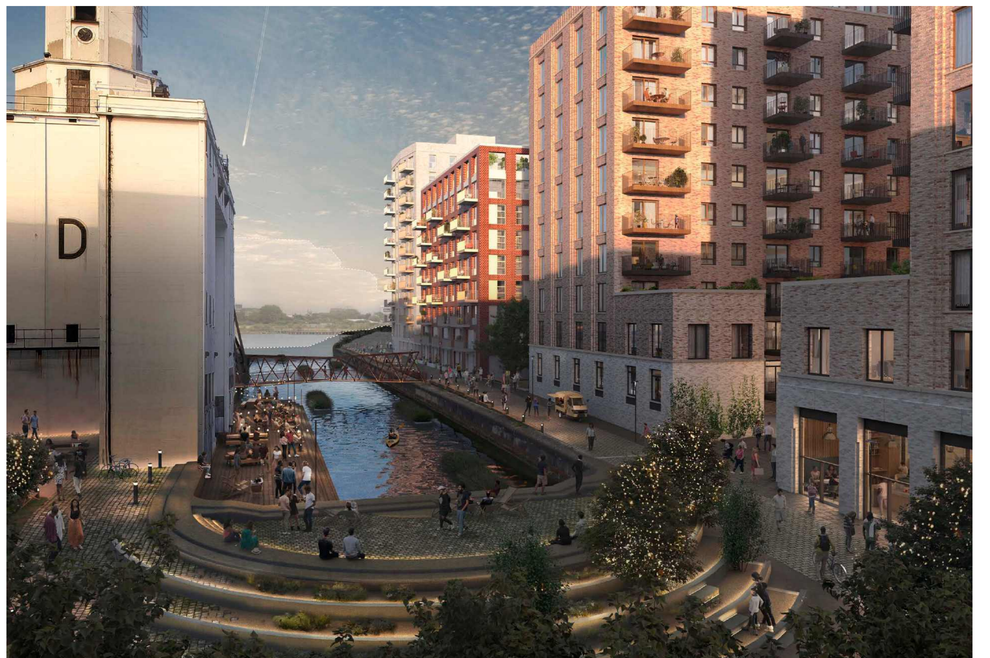
The above Computer Generated Image (CGI) shows detail of consented Phase 1 with Silo D.
