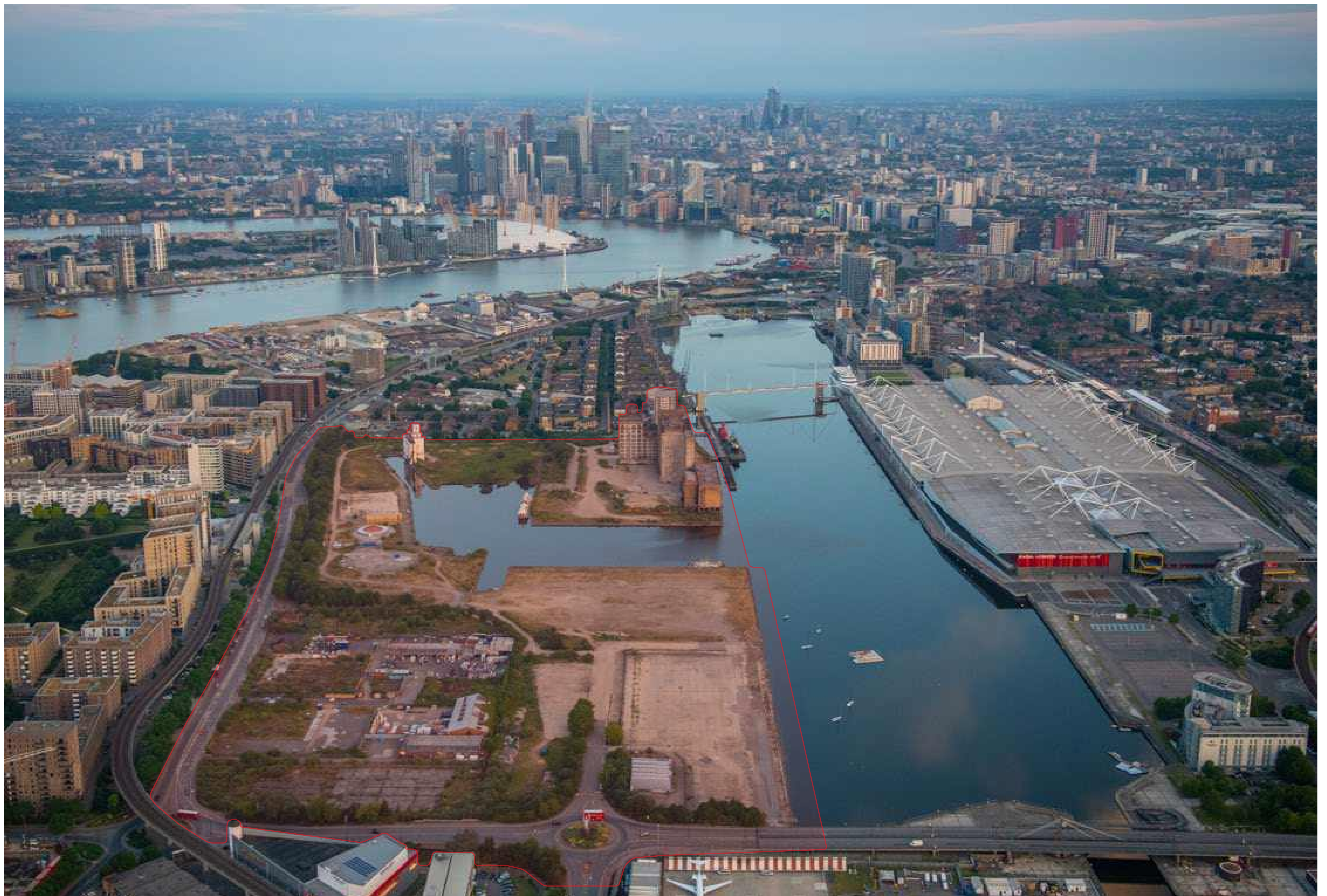
This birds-eye view shows the Silvertown site (outlined) by the Royal Victoria Dock and opposite the ExCeL. The Greenwich O2 and Canary Wharf can be seen in the background.
