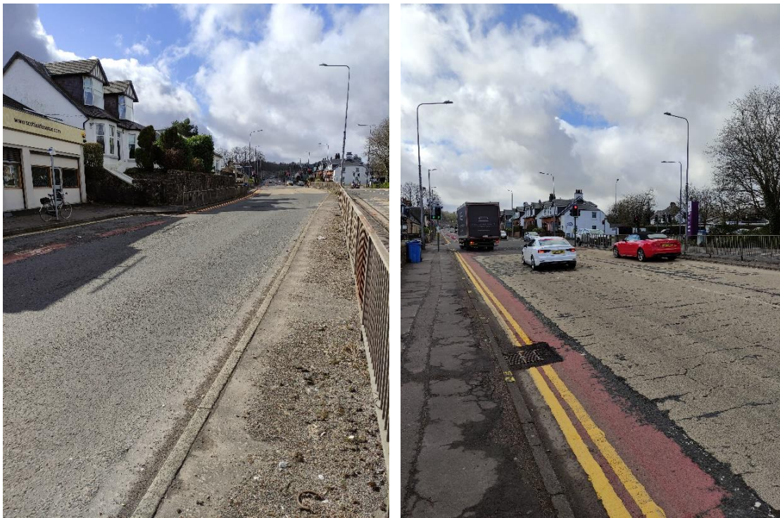
Plate 4: Removal of temporary measures at Mearns Cross
