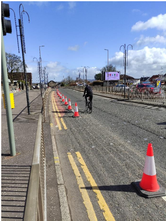
Plate 2: Substandard cycle lane widths and potential hazards (ironwork and cones)
