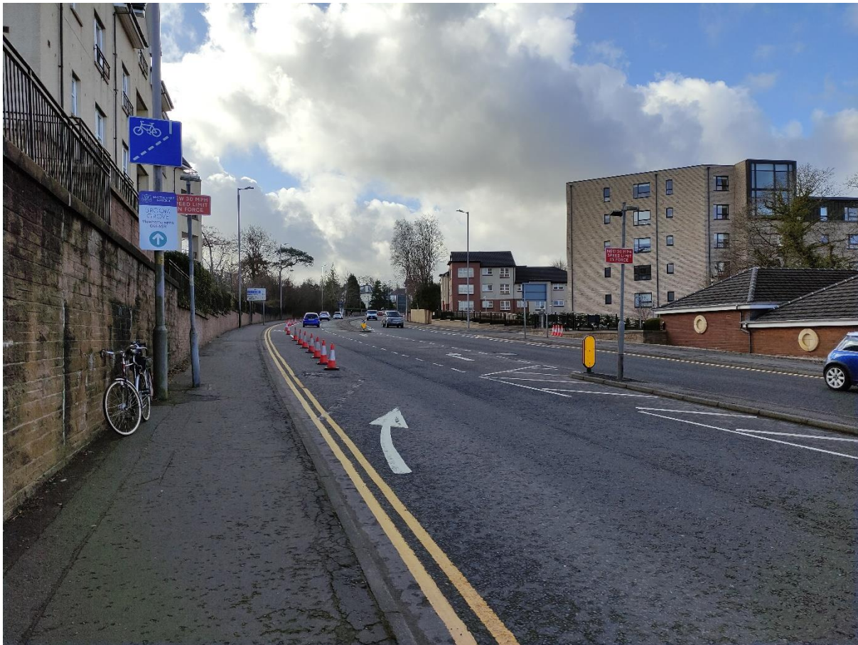
Plate 3: Temporary advisory signage to support speed limit reduction
