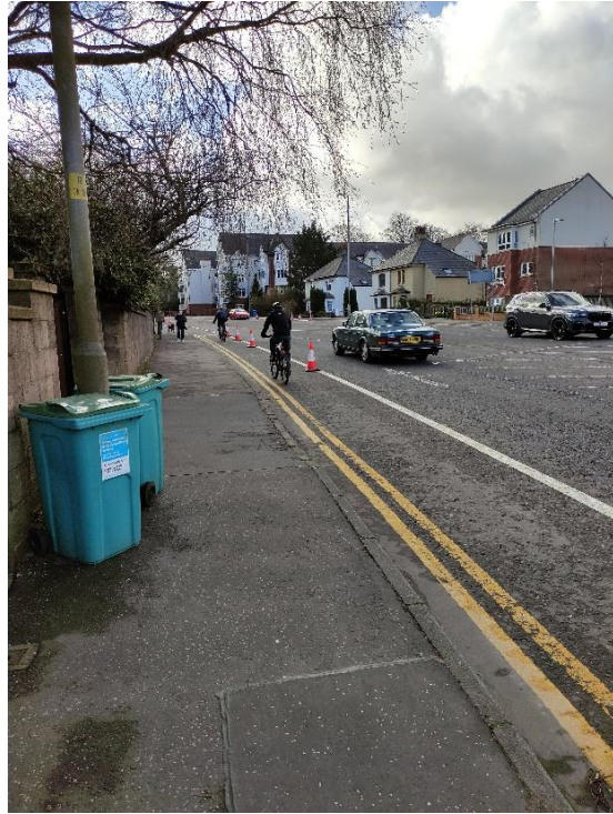
Plate 5: Example of regular 'breaks' in segregation (generally at driveways and junctions)
