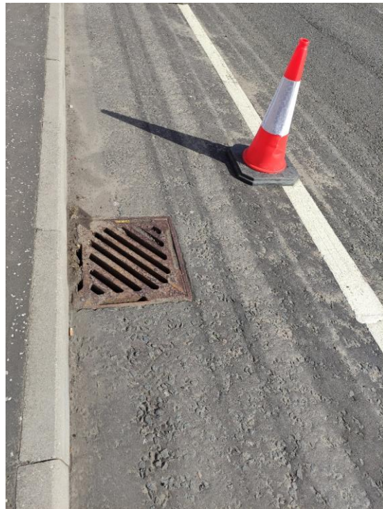
Plate 2: Substandard cycle lane widths and potential hazards (ironwork and cones)
