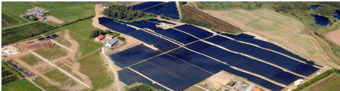
Figure 18: An aerial view of the Silkeborg solar thermal array in Denmark
