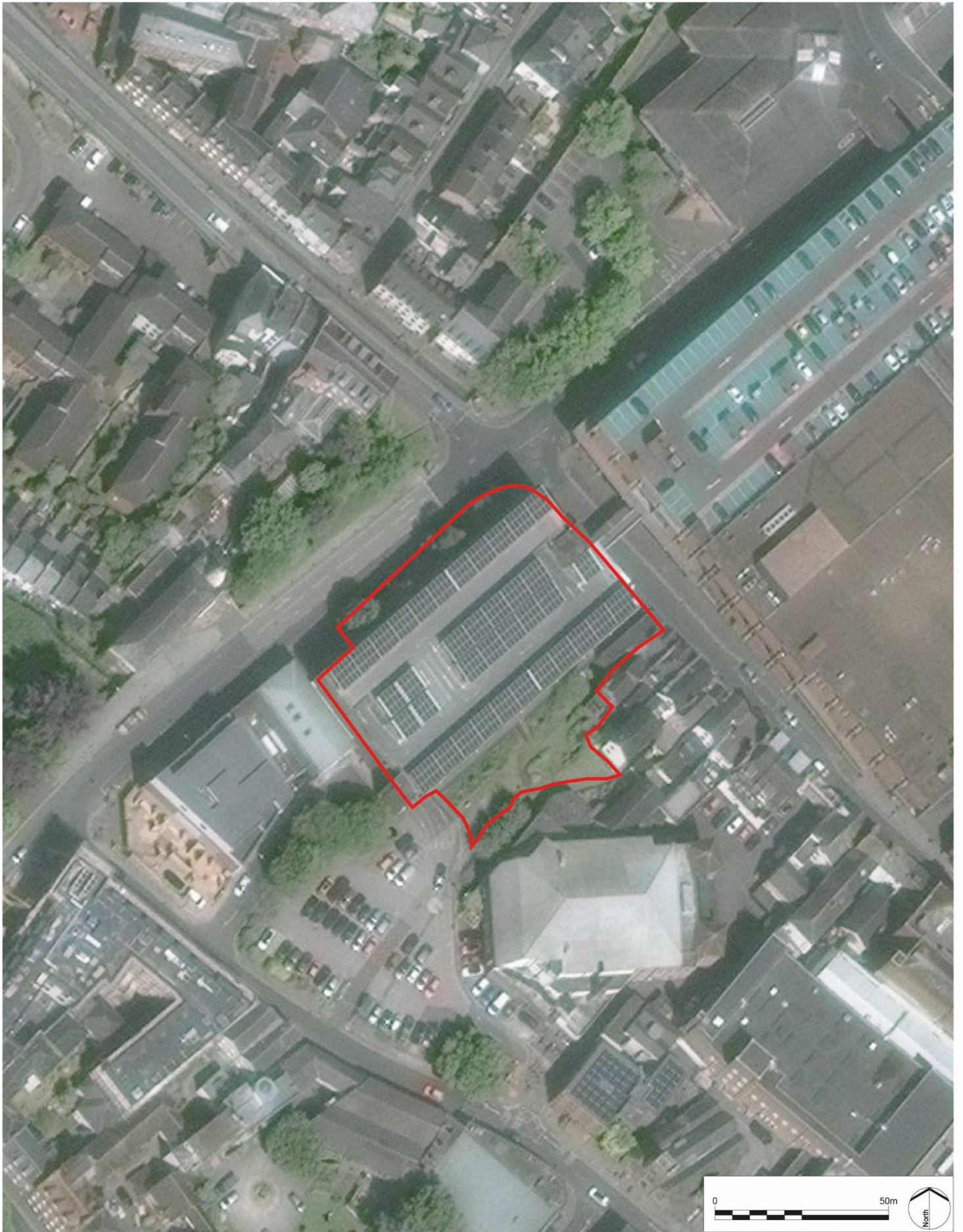
Mary Arches Car Park Total Site Area: 0.28 Ha
