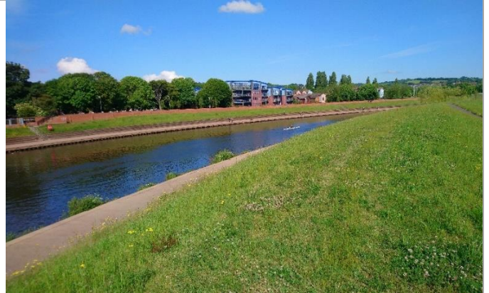
View across overflow channel towards hill backcloth.
