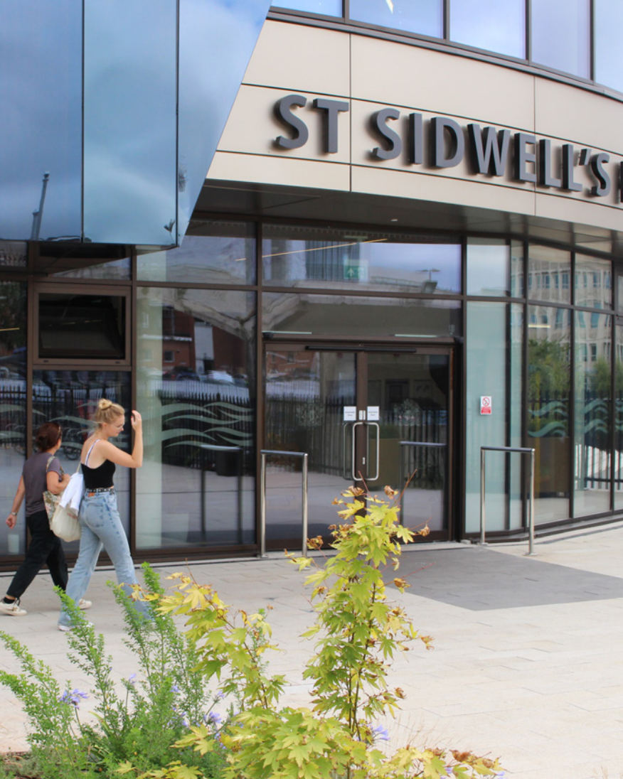
St Sidwell's Point is the UK's first Passivhaus pool demonstrating the City's commitment to leading the way in net zero carbon, promoting innovation and placing Exeter on the global stage
