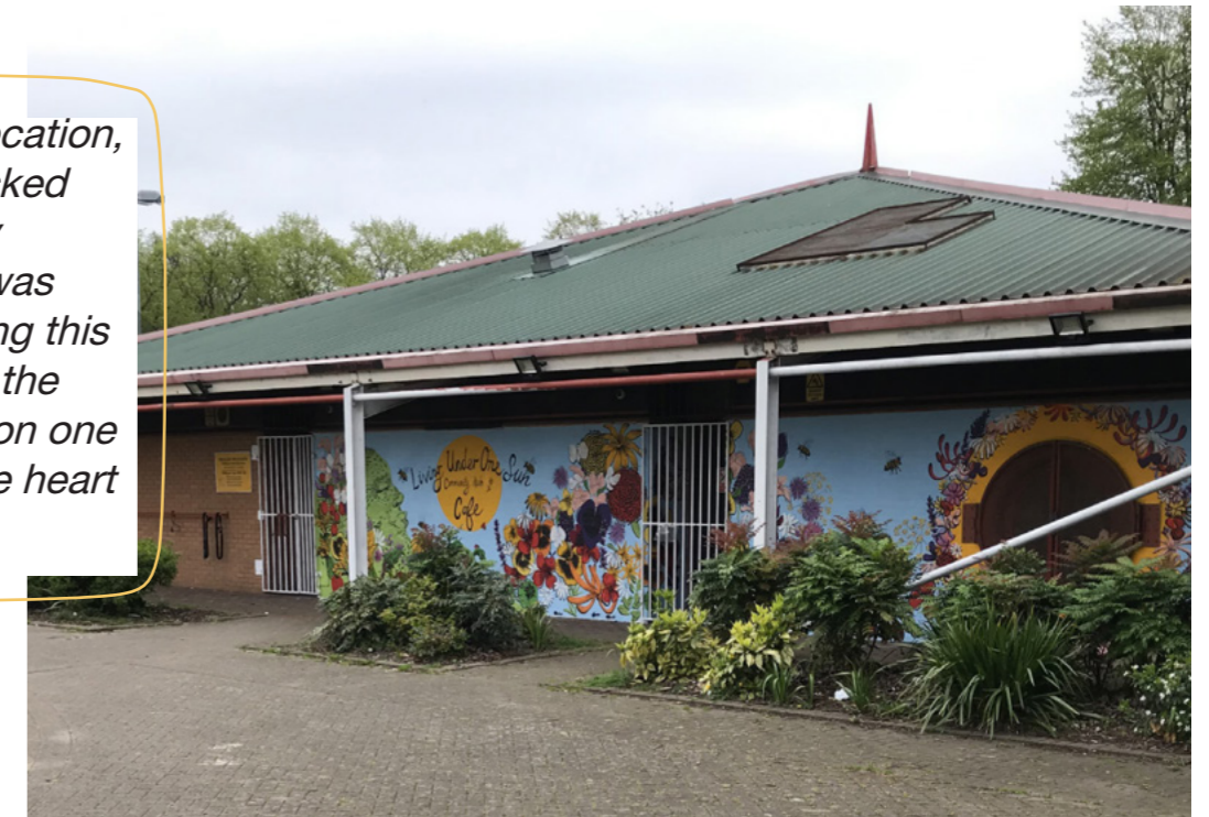
Pavilion building, Down Lane Park.
