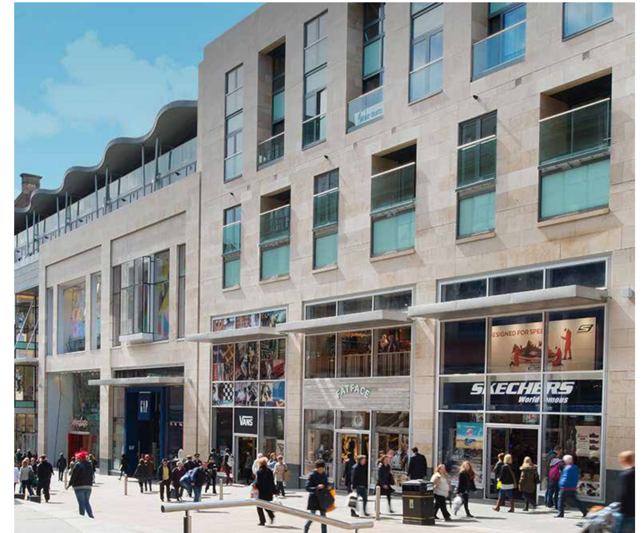
Atlas, 185-221 Buchanan Street. A multi award-winning retail and residential area developed and owned by Landsec, completed in 2013.
